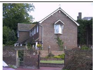
Figure 5- Station Road (south side)
