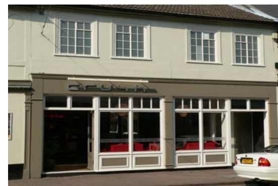
Plate 3– New paired, mirrored design on a two property knock-through to form a public house frontage, with adjacent listed building
