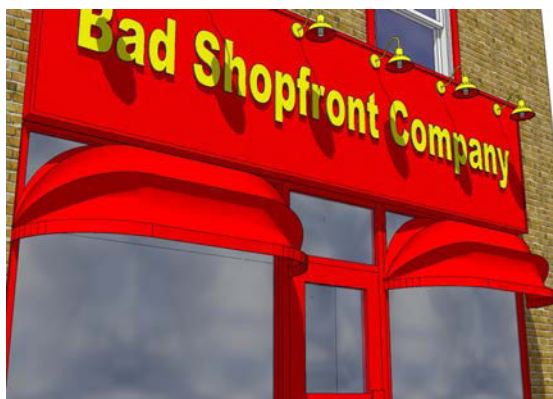
Figure 15– Fixed canopies are often inappropriate.
