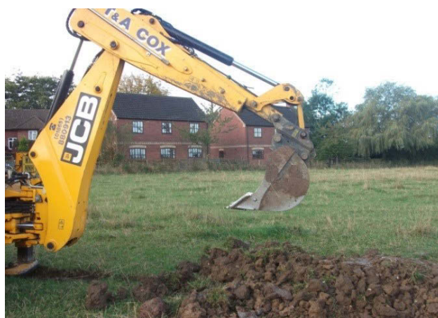
Figure 4 – Example Trial Pit
