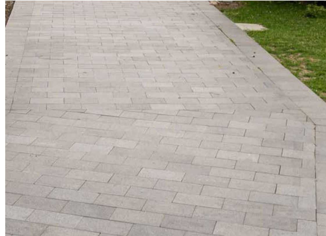
Figure 88. Porous Granite for public realm next to the River Darent 300 x 100mm
