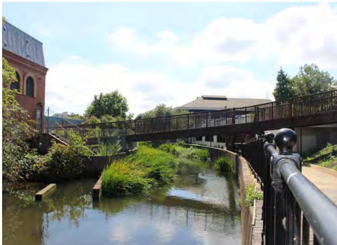
Figure 31. Site photo of the River Darent in Dartford Town Centre
