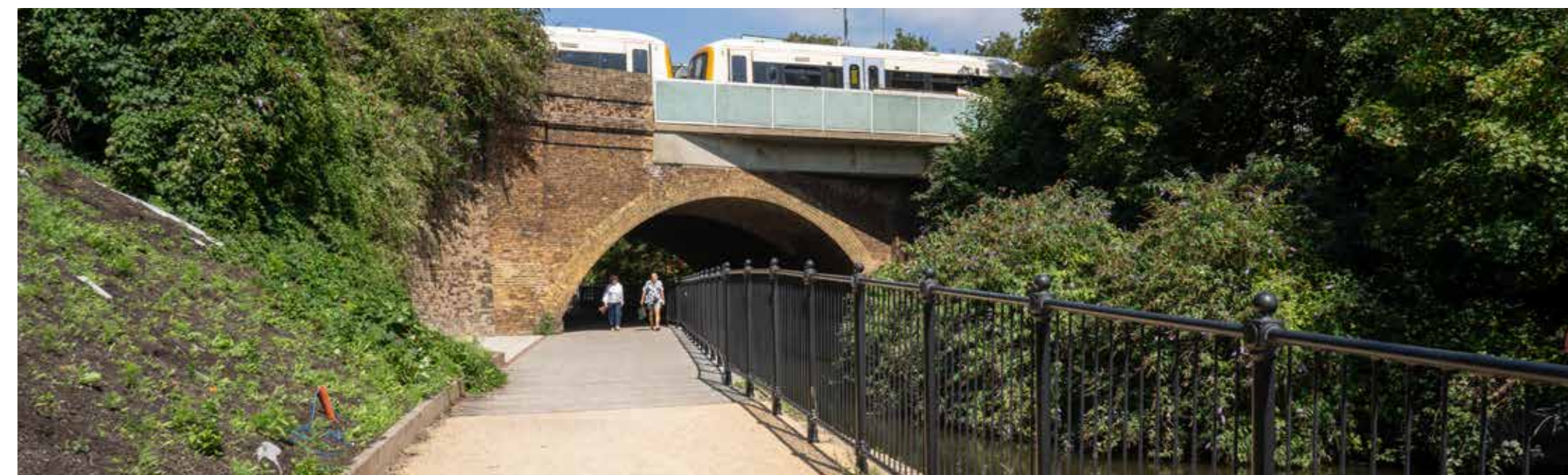
Figure 61. Existing black metal railings
