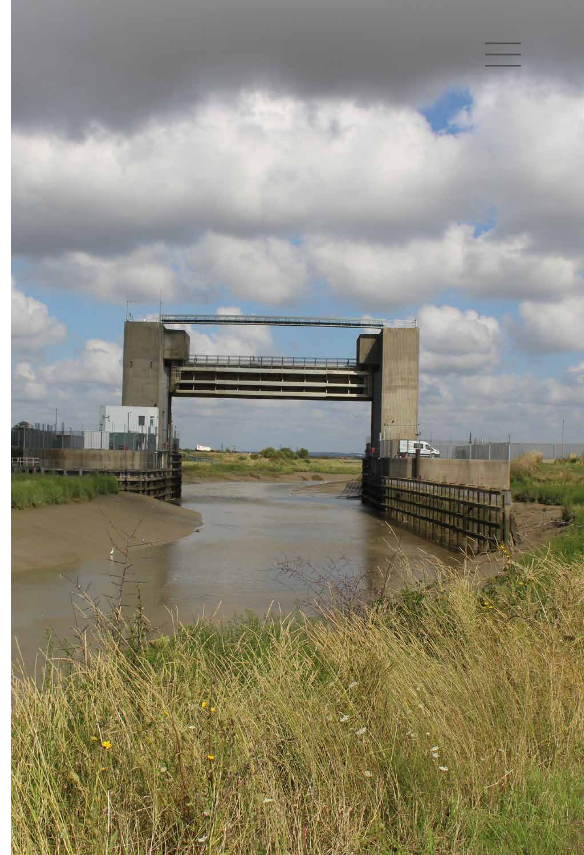
Figure 119. Dartford Creek Barrier
