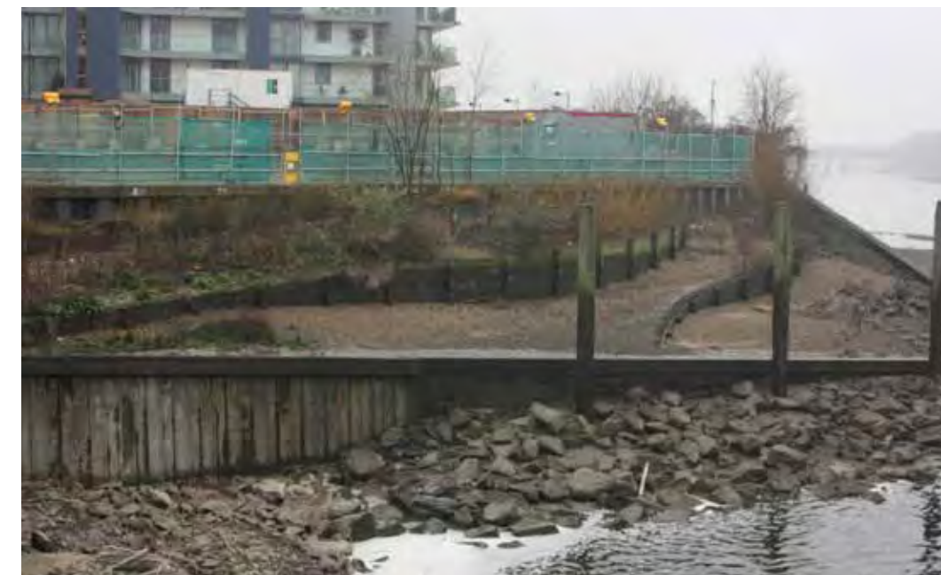
Figure 53. Cut down wall with installed terracing
