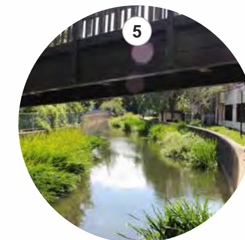
5. River in Dartford Town Centre lined by walls
