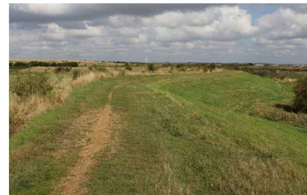
Figure 42. Site photo existing Dartford Marsh embankment
