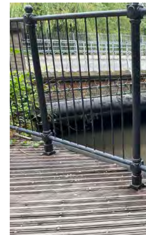
Figure 99. River edge black metal railings
