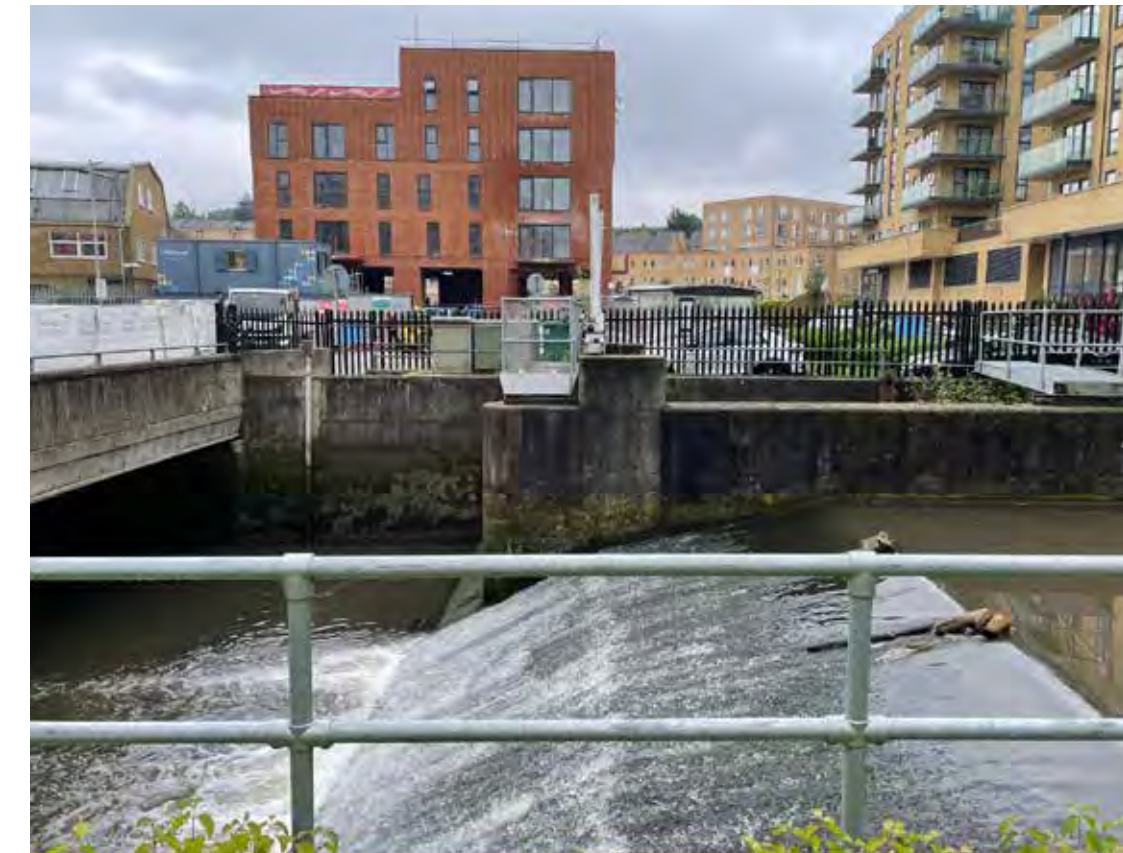
Figure 65. Site photo of the Wellcome Sluice
