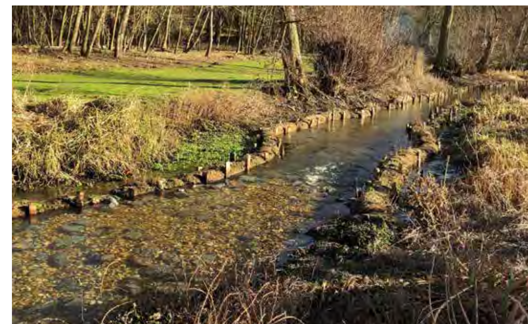
Figure 80. Brushwood mattresses restore river edge
