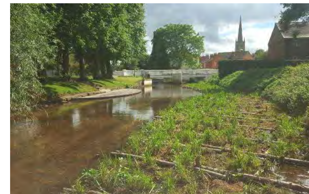
Figure 81. Angle of slope decreased using brushwood mattresses
