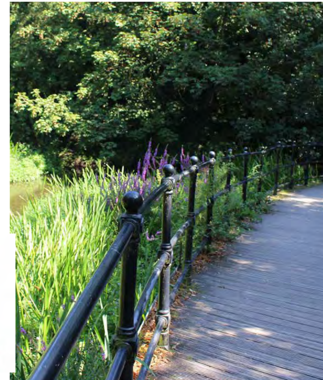
Figure 69. Site photo of the river in Central Park
