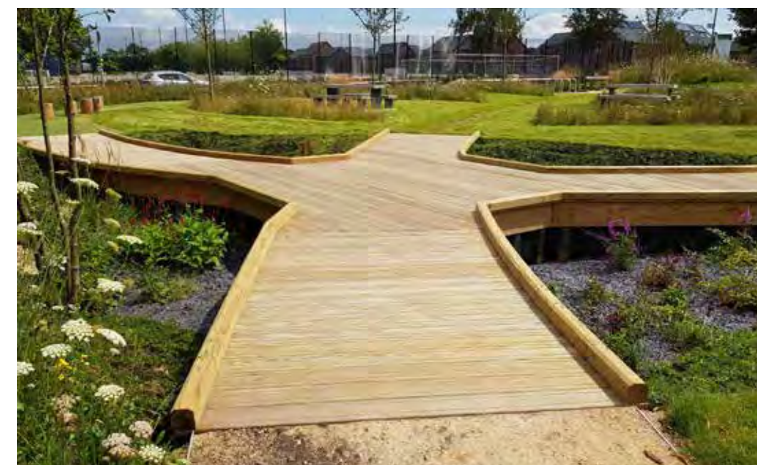
Figure 76. Timber boardwalk over a gravel planted attenuation basin
