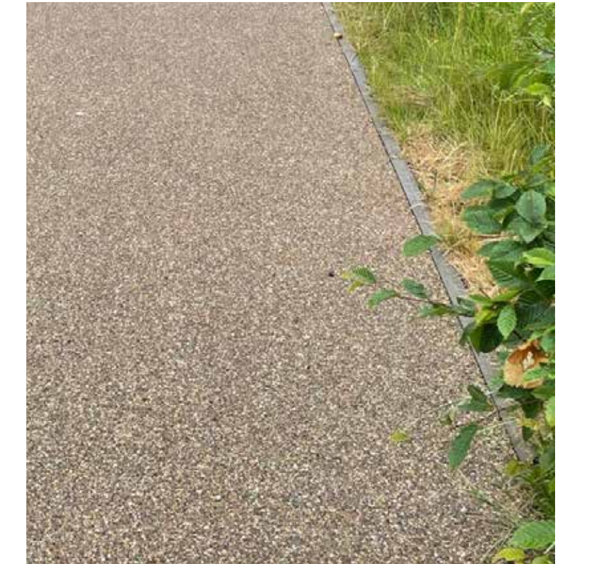
Figure 93. Buff coloured Tarmac for urban sections of Darent Valley Path
