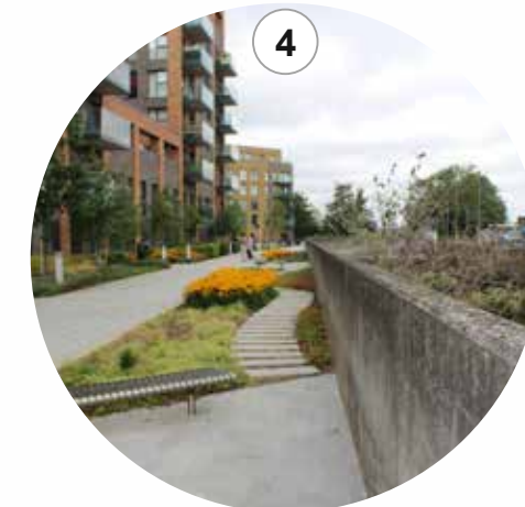
4. New public realm alongside the river in Dartford Town Centre
