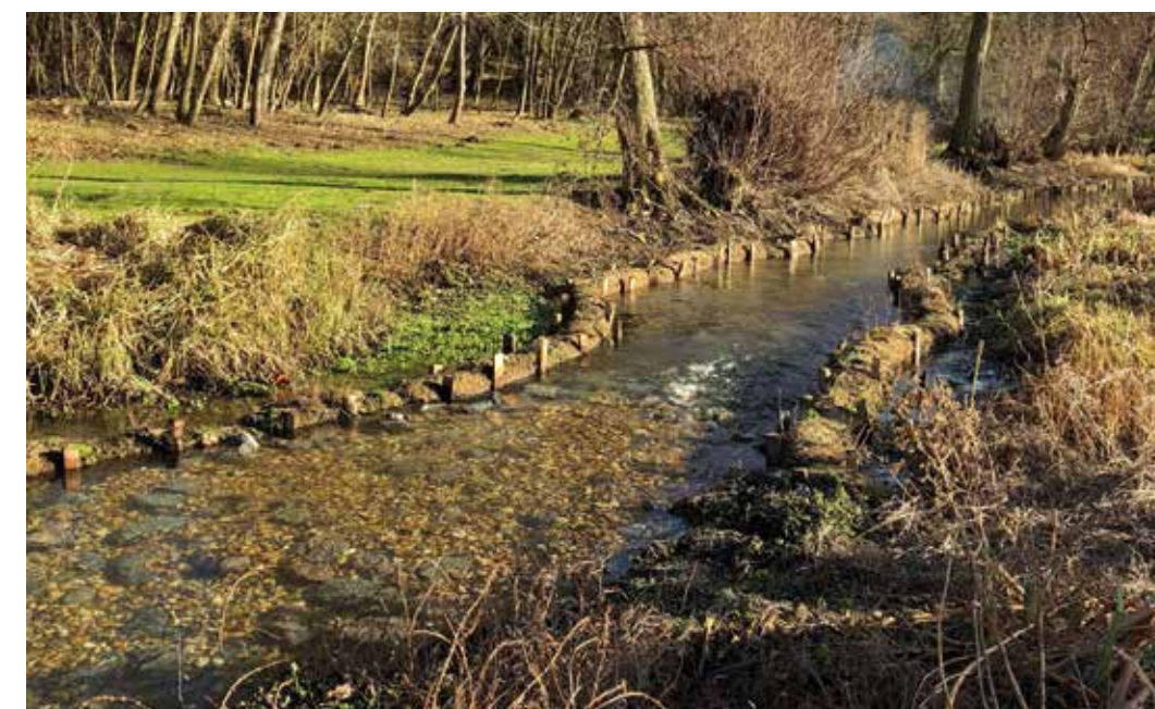
Figure 80. Brushwood mattresses restore river edge
