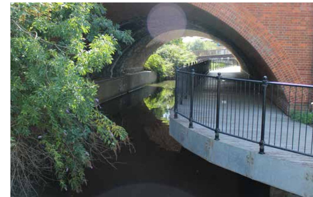
Figure 64. Site photo existing railing character
