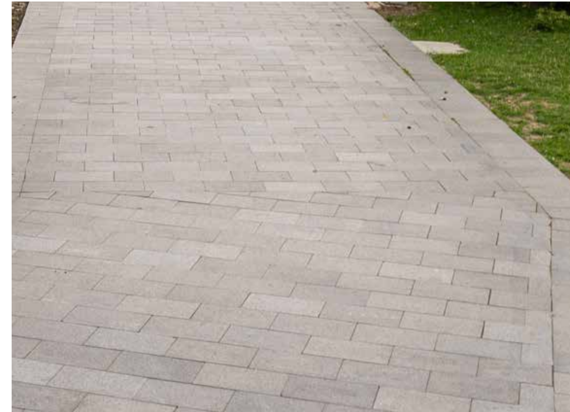
Figure 88. Porous Granite for public realm next to the River Darent 300 x 100mm
