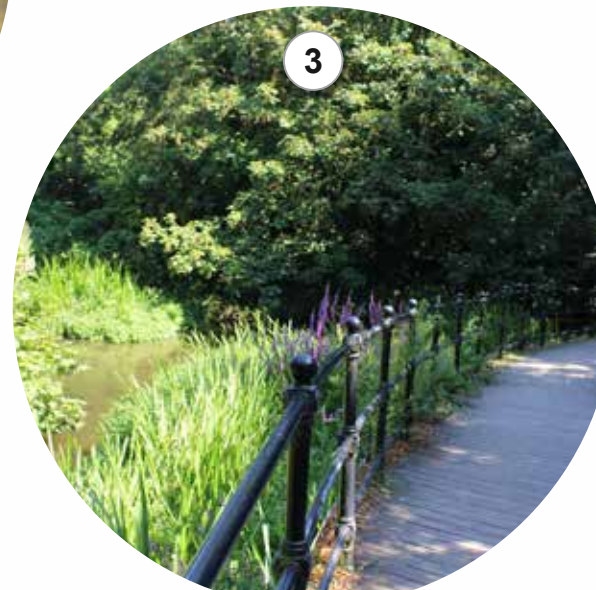
3. Timber deck edge to river
