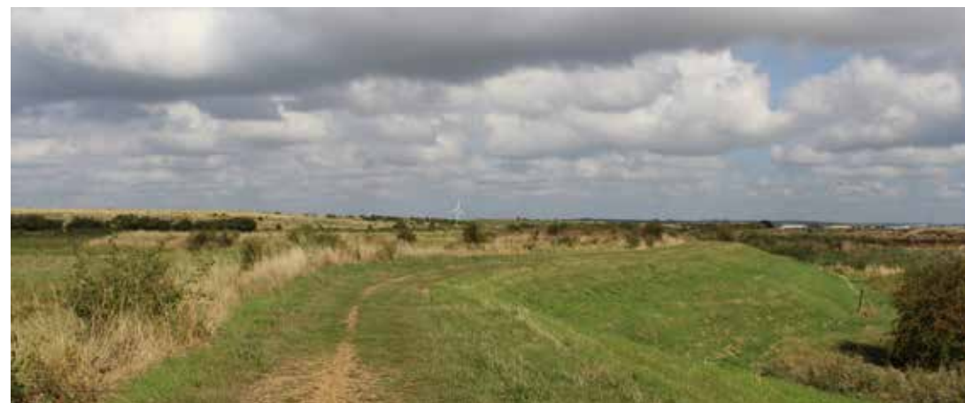
Figure 23. Existing embankment in Dartford Marshes
