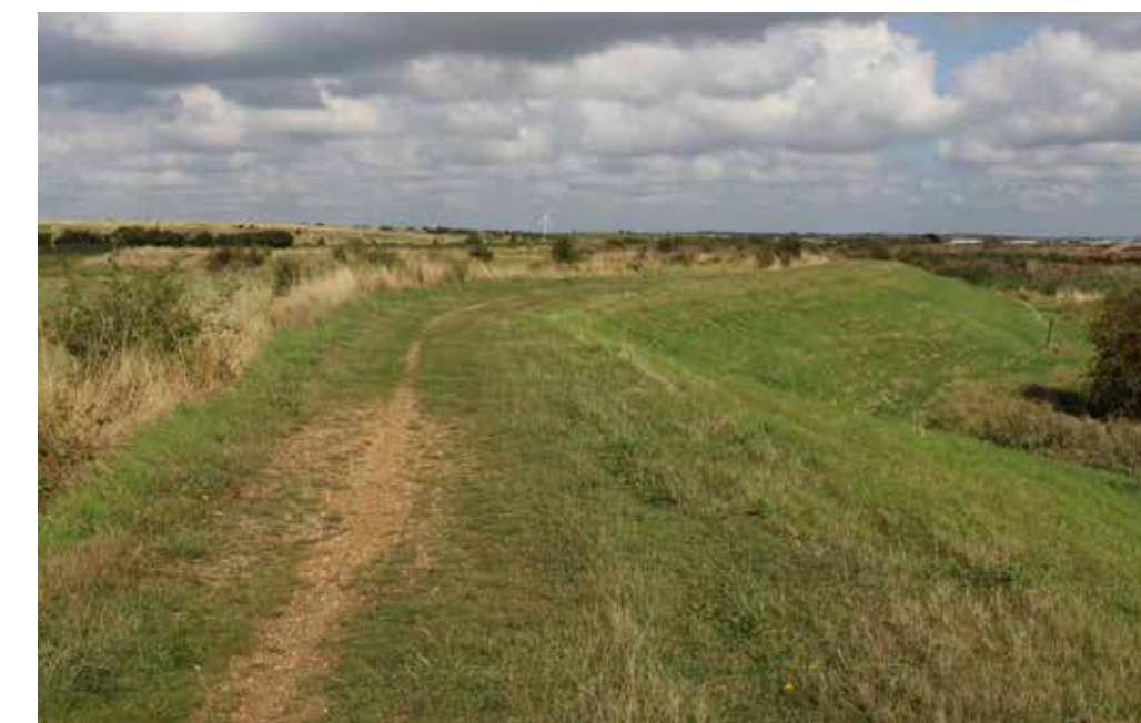
Figure 42. Site photo existing Dartford Marsh embankment
