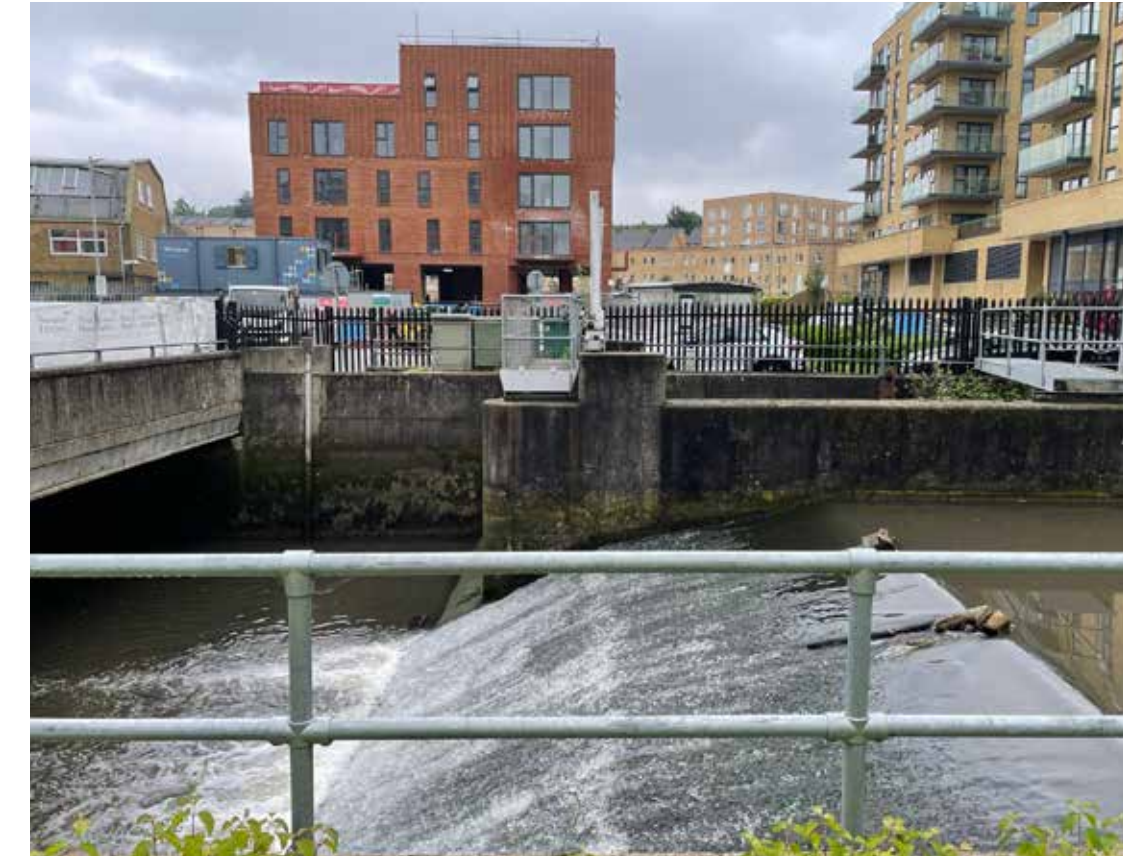
Figure 65. Site photo of the Wellcome Sluice
