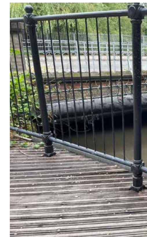
Figure 99. River edge black metal railings
