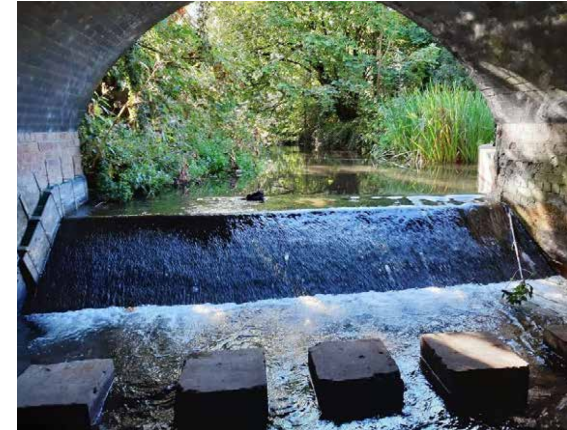
Figure 68. Site photo of the Princess
