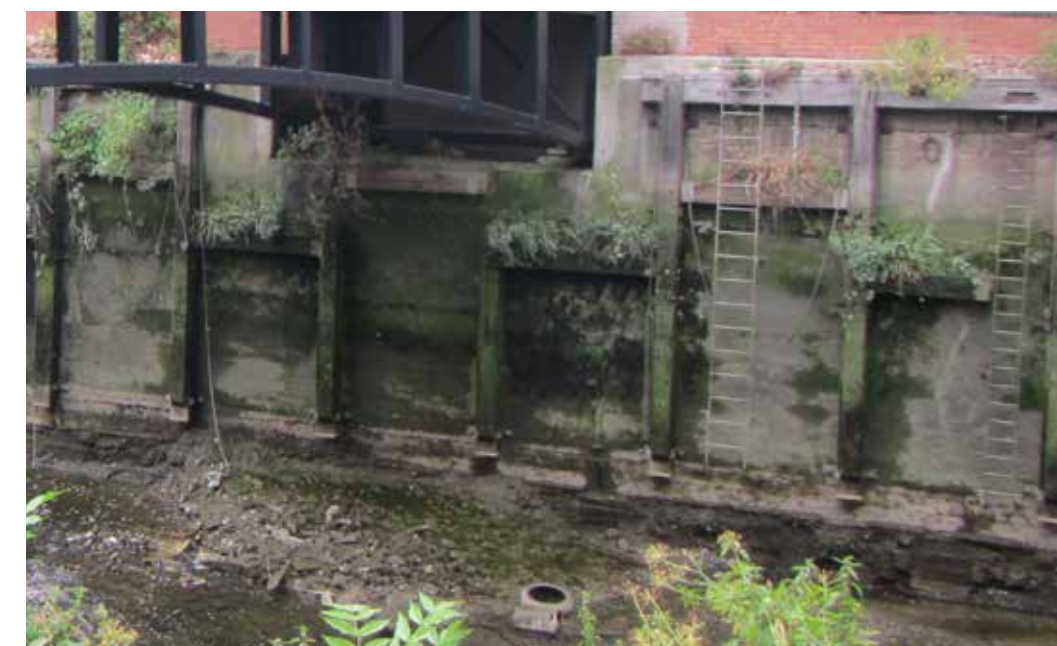
Figure 58. An example of an ecological treatment to a vertical river wall
