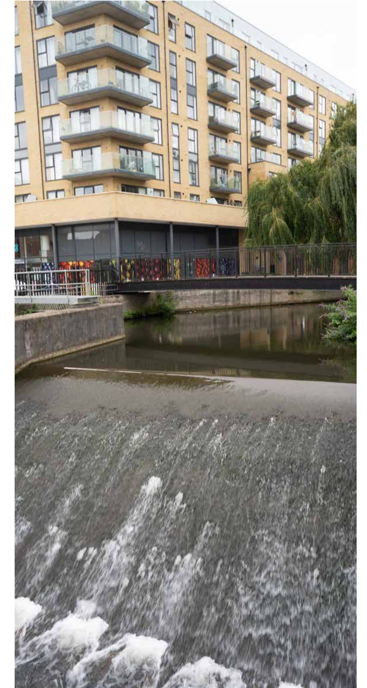
Figure 67. Site photo of the Wellcome Sluice
