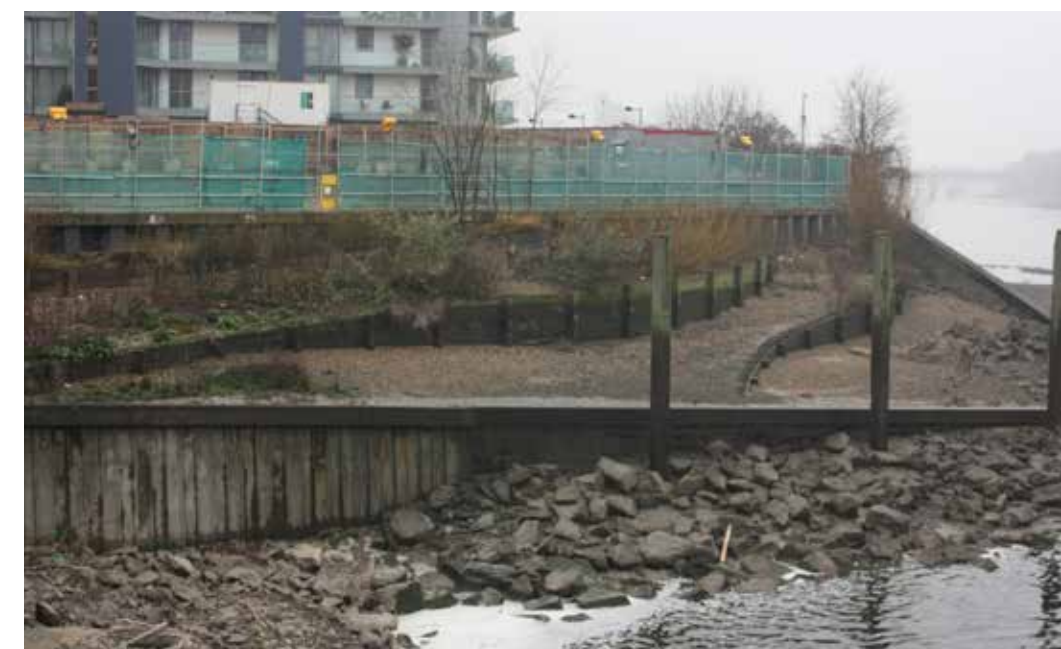
Figure 53. Cut down wall with installed terracing
