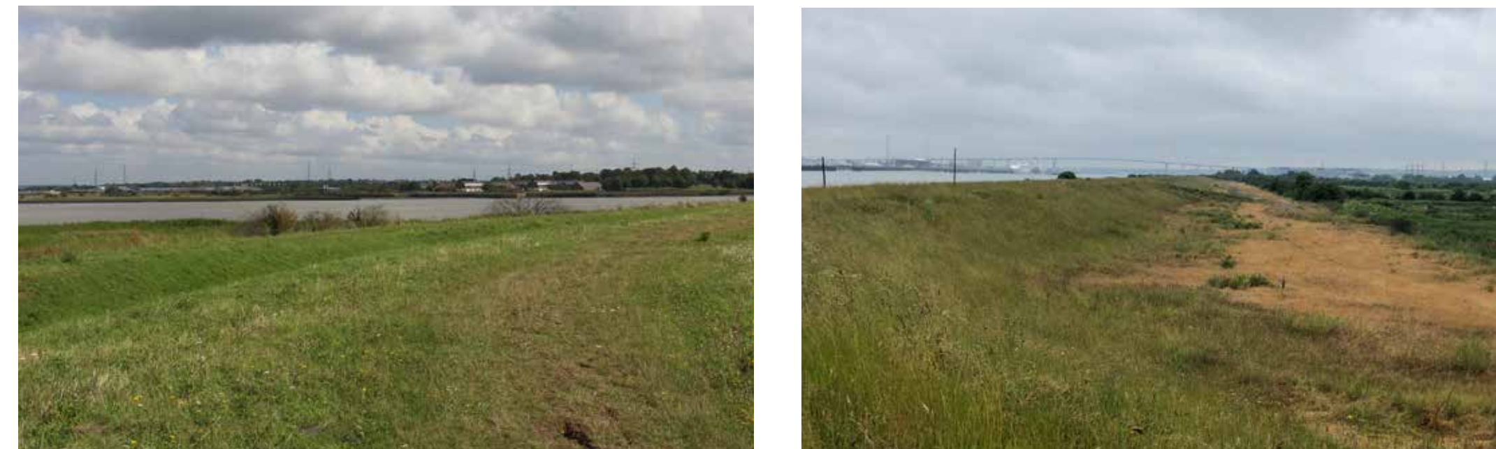
Figure 39. Site photo existing Thames edge flood defence embankment
