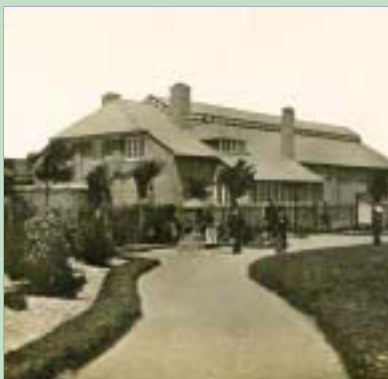
Drill Hall, Central Park
